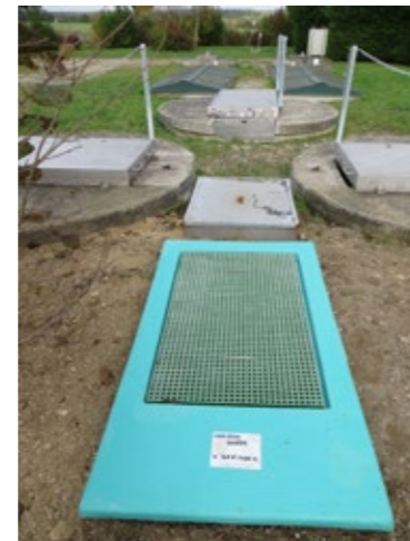
Station d'épuration Courson-Monteloup
